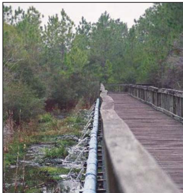
Figure 2. Emerald Coast Utility Authority Bayou Marcus Wastewater to Wetland Treatment System
